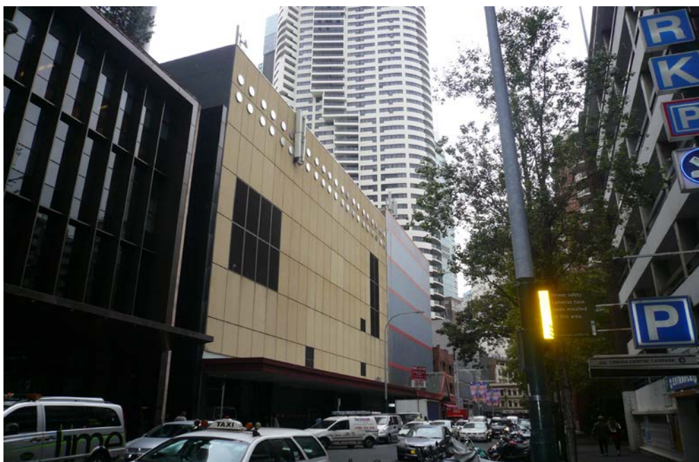
Figure 4 – Kent Street Elevation of the Existing Building
