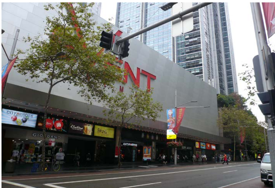
Figure 3 – George Street Elevation of the existing Building
